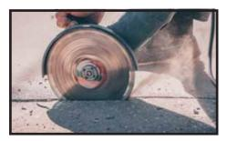
4. Put the mounting bracket on stone or cement surface, cut the mounting bracket along the dot line with grinder if you don't have enough installation room, which is only for your reference, cutting varies based on your actual application
